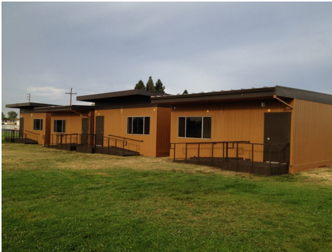
Interim Housing Portable Classrooms
